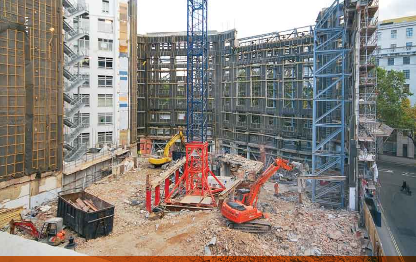
▲ Temporary bracing supports the 100-year-old façade of 1-5 Kingsway to allow for demolition to the single basement level.
